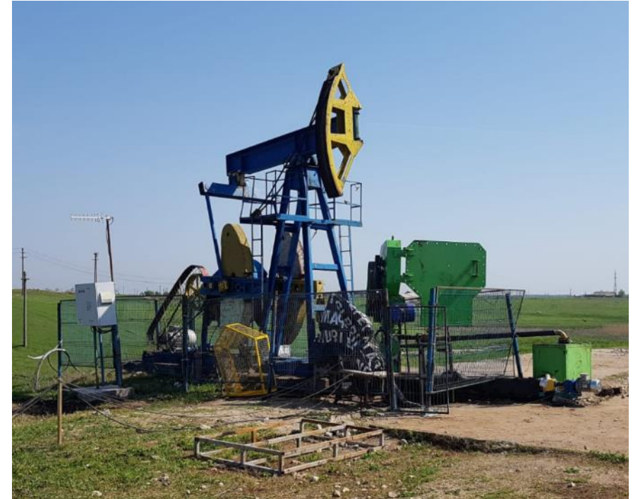
Conventional Sucker Rod Pump (Blue & Yellow) besides the HOOS Unit (Green) that has replaced it
